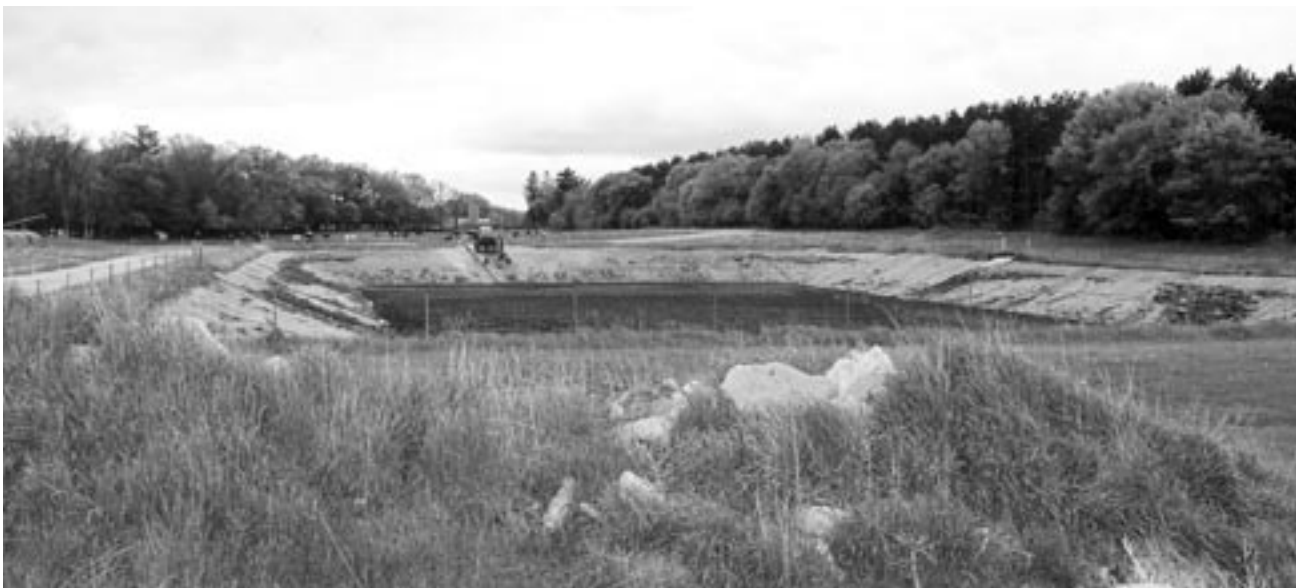
A lined manure storage basin at one Minnesota dairy.
